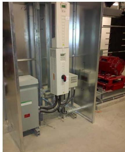
*Lineator AUHF and VSD on chilled water pump*
